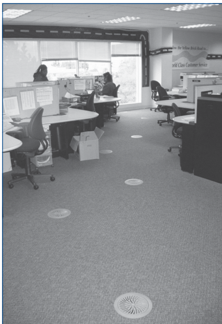
Figure 4. Typical interior swirl diffuser layout.
